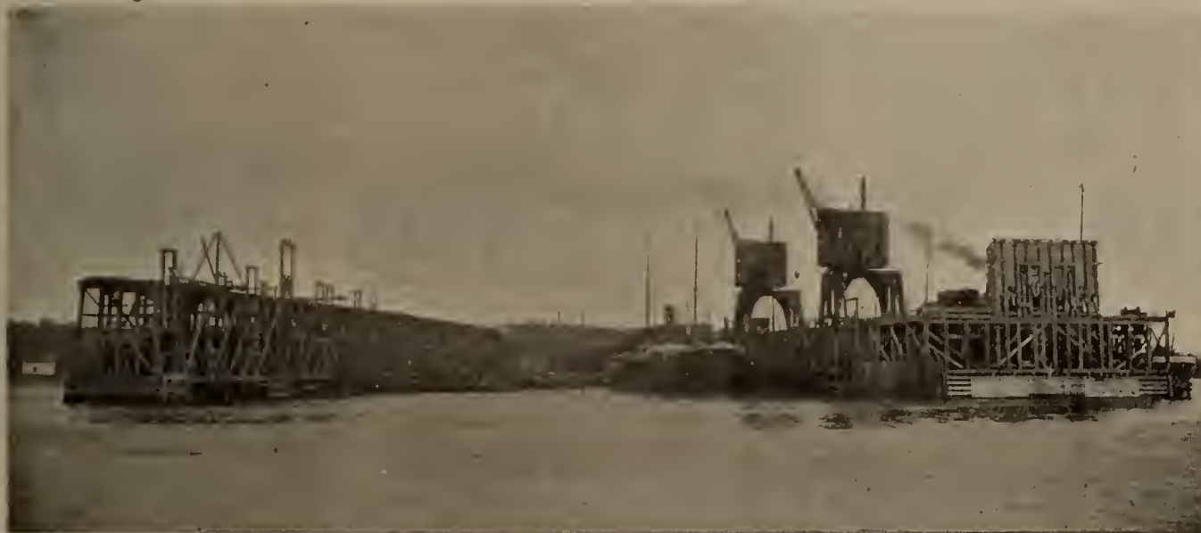
International Shipping Piers of the Dominion Coal Co. Limited, at Sydney, C.B.
